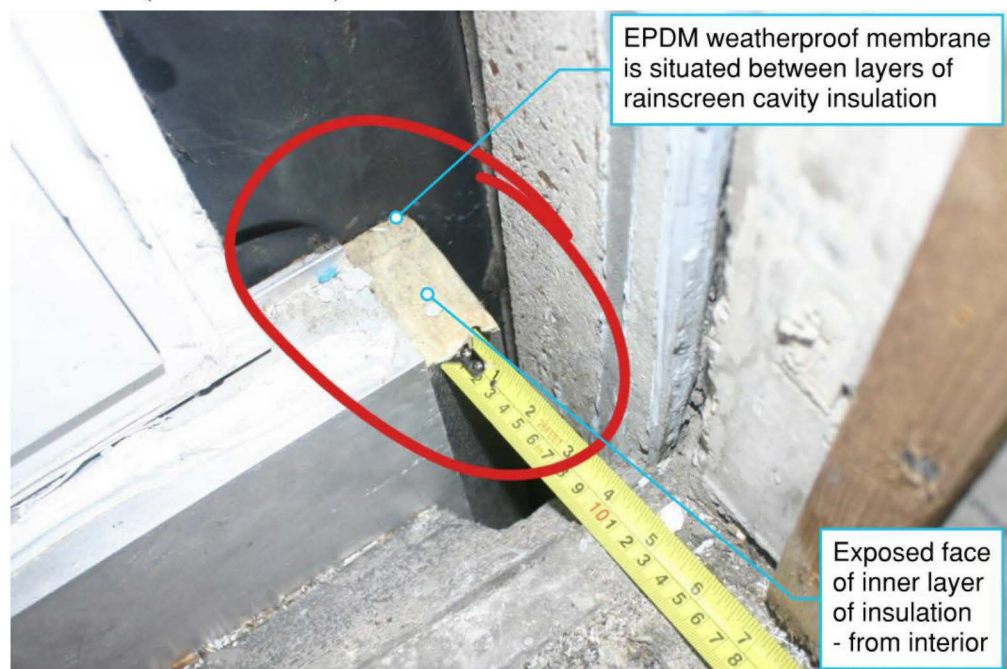
Figure 8.31: Rainscreen cavity insulation visible from interior due to EPDM weatherproof membrane bonded between insulation layers, in close proximity to gap and EPDM weatherproof membrane (Flat 13)
