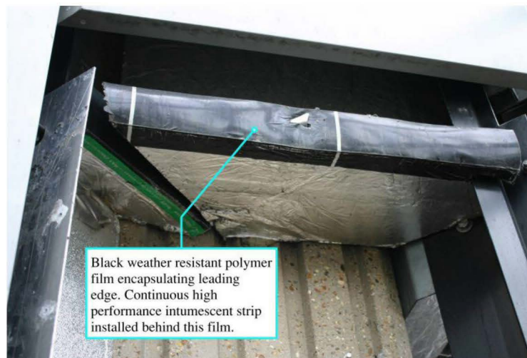
Figure 8.45 Position of black weather resistant polymer film and continuous high performance intumescent strip
