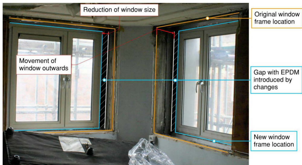
Figure 8.24: Photograph showing changes and how they introduced gaps around the window frames (Flat 13)
