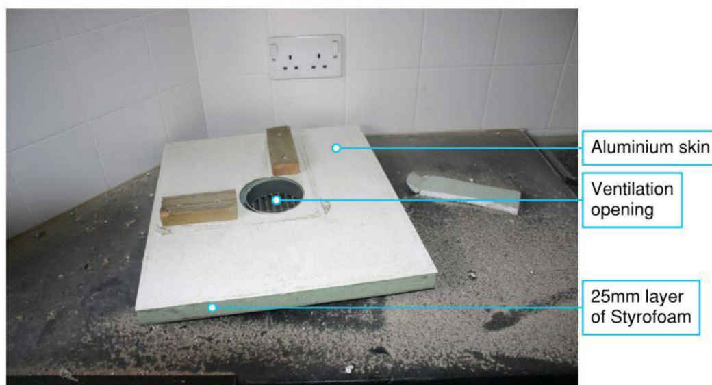
Figure 8.73: Window insert insulating core panel removed from glazing system. Flat 10 Kitchen (however this window insert was present for every flat as per the Harley specification (HAR00008991)).
