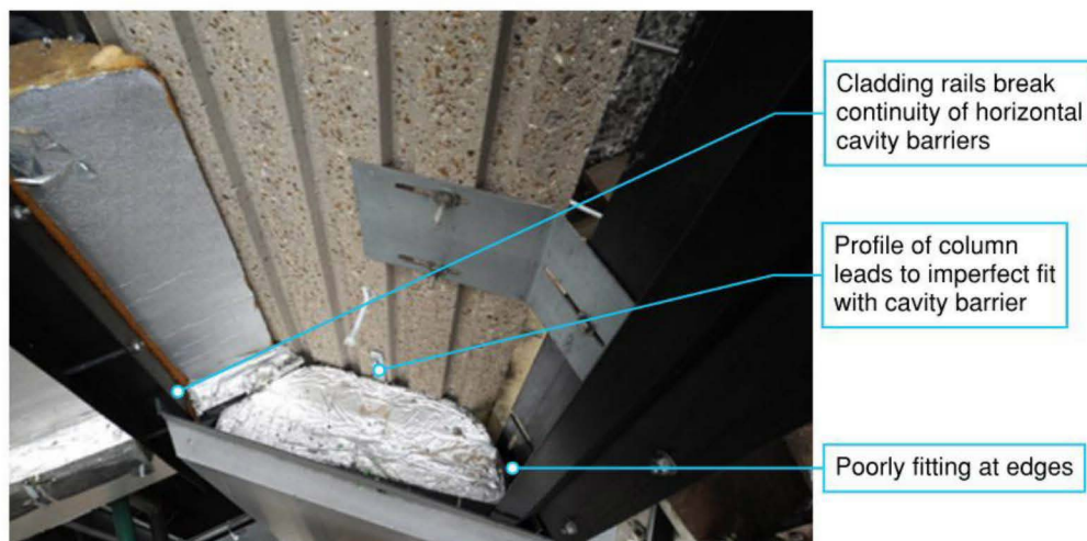
Figure 8.44: Junction of column and spandrel horizontal cavity barrier. External of Flat 12.
