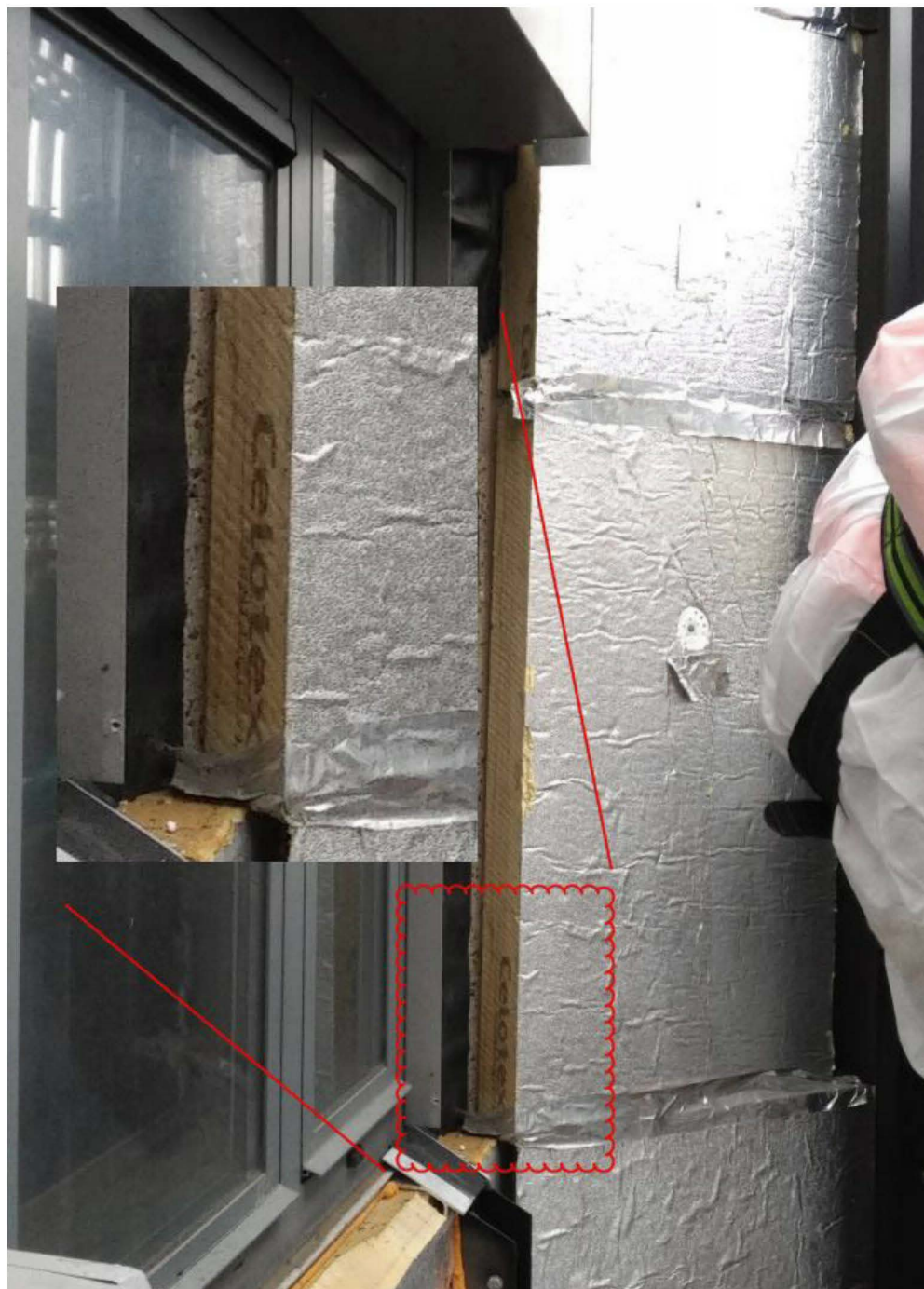
Figure 8.37: Evidence of Celotex in place as part of the external wall
