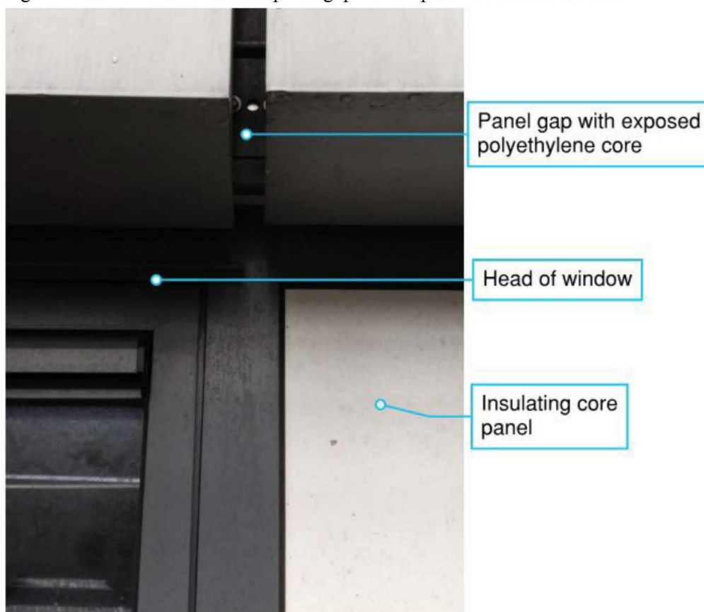
Figure 8.66: Panel gap in spandrel rainscreen cladding panels at head of window. Flat 10.
