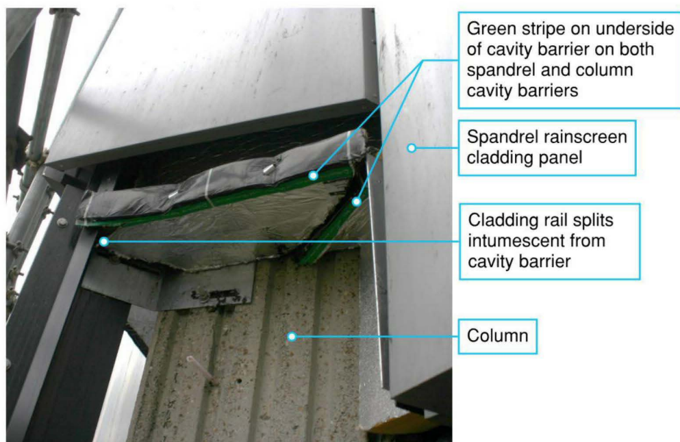
Figure 8.47: Cavity barriers installed onsite with green stripe on the bottom face of the cavity barrier, as well damage leading to the intumescent strip separating from the cavity barrier. External of Flat 12.
