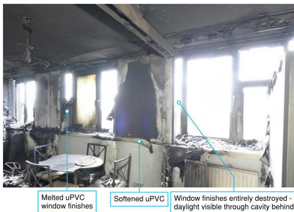
Figure 8.32: Post-fire condition of window finishes in fire damaged flat (METS00017068) (Flat 93, Level 12)
