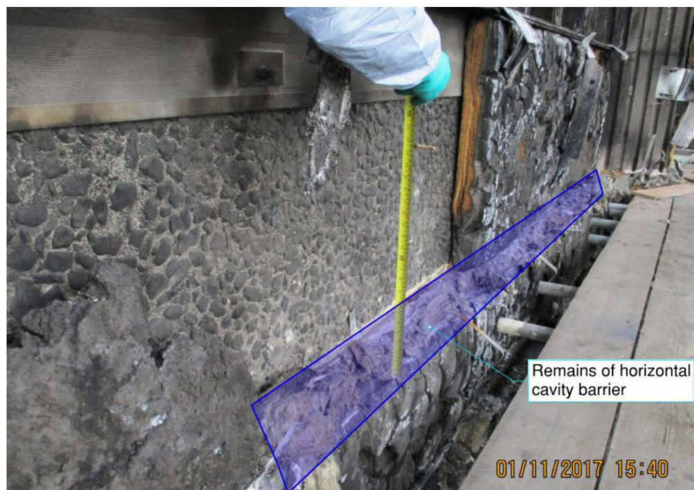
Figure 8.42: Evidence from site of position of cavity barrier (Flat 16, Bedroom 2)
