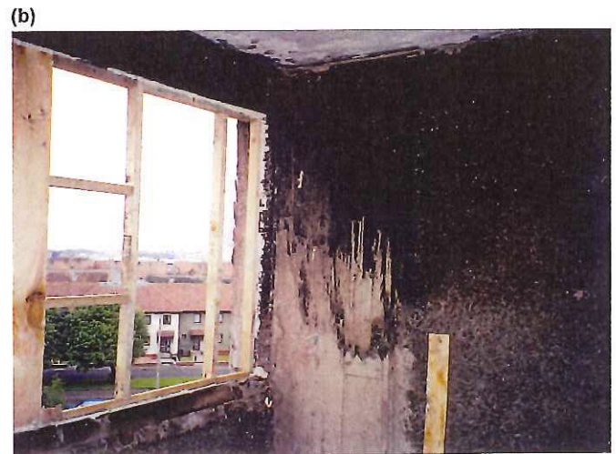
Figure 4: (a) Fire breakout from a post-flashover room on a masonry facade, (b) result of the flashover
