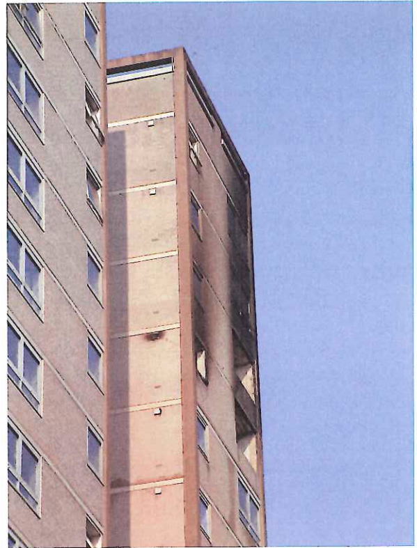
Figure 5: Fire damage
