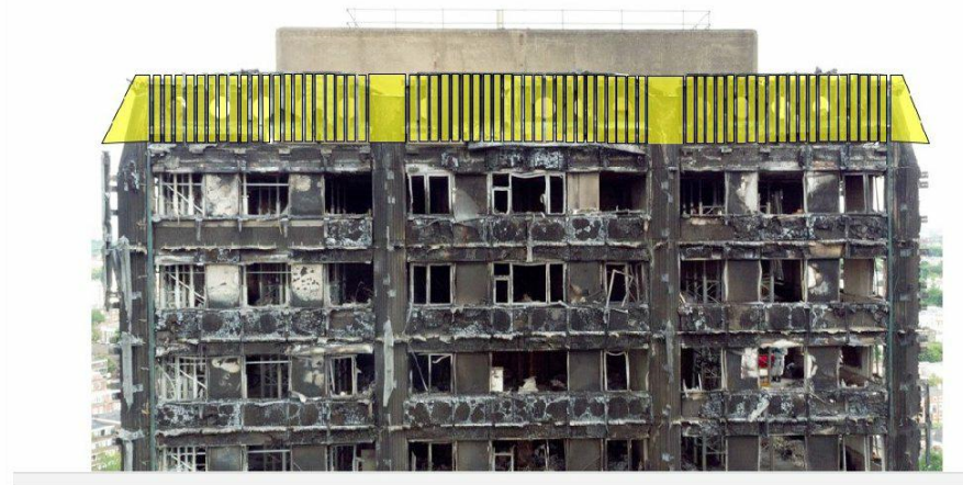
Upper floors of Tower showing extensive loss of cladding, insulation, and window infill panels MET00004491
