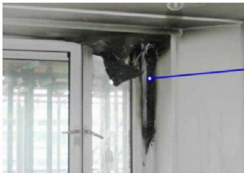
Figure 10.52: Burned uPVC frame in Flat 15
